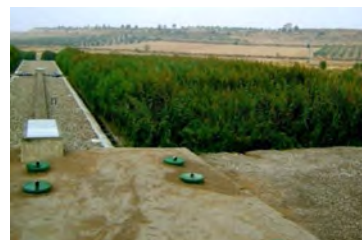
Centralized STP based on CWs in Czech Republic
