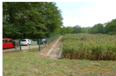
Full-Scale CW facility for a Village in Spain
