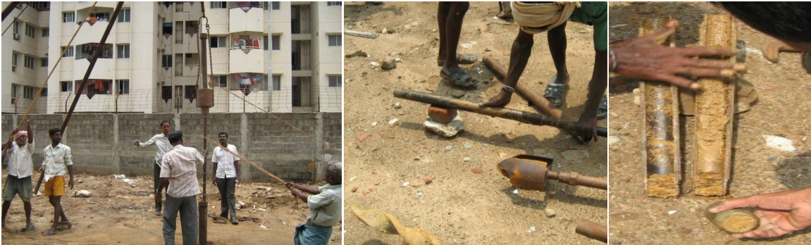
Plate 1 SPT test in progress
