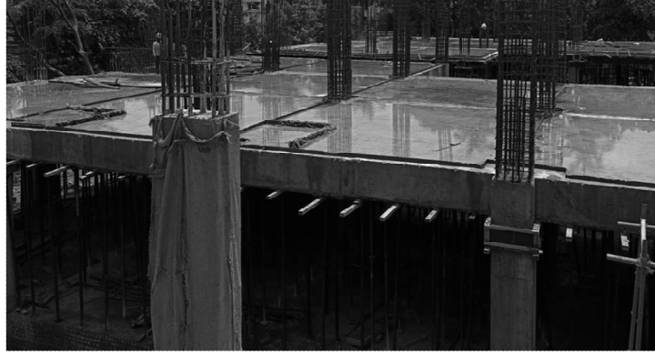
FIG.6 CASTED IWSB FOR PSEUDO SUNKEN ARRANGEMENT
