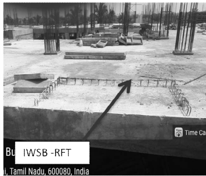
FIG.3 & 4 REINFORCEMENT FOR IWSB (BEFORE FINISH)
