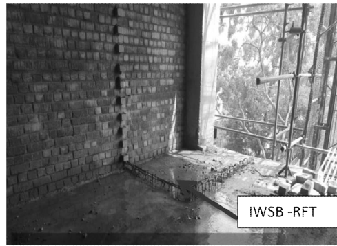
FIG.3 & 4 REINFORCEMENT FOR IWSB (BEFORE FINISH)
