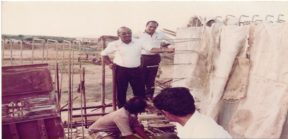
Checking the reinforcement of the deck at the Athipattu Bridge during the period of May, 1991
